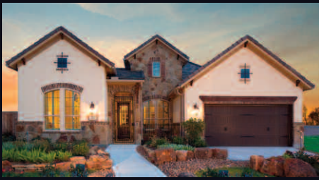
Volume Builder Garden Home/Patio Home of the Year TRENDMAKER HOMES
